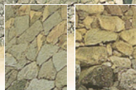
Otoshi-Tsumi Gobou-Tsumi (A method of piling stones)
